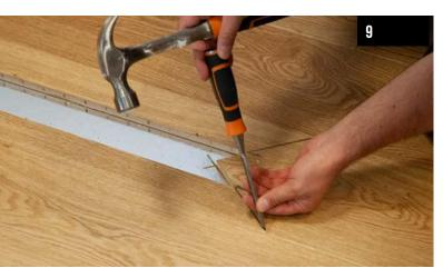
Use a chisel or multi-tool with wood saw blades to cut the uncut corners of the damaged board. When cutting, be careful not to damage the adjacent boards.
