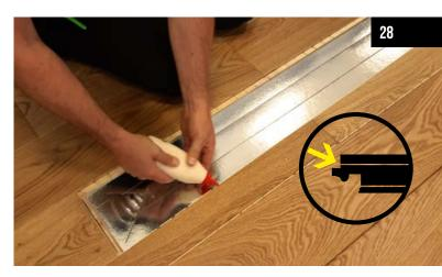
Apply waterproof carpentry glue to the outer part of the long edge of the tongue of the adjacent plank.
