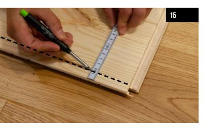
Turn the board over and mark a line on the bottom layer from the side of the longitudinal groove along its entire length at a distance of 15 mm (9/32") from the edge.
