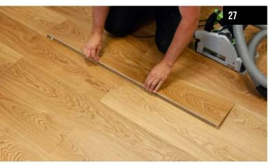
Make an attempt to fit the board. In case the board is too tight of a fit in width or length, correct the new plank with sandpaper or a small plane. Check to see if the board fits; now remove the replacement board and then insert the previously removed 5Gc insert.
