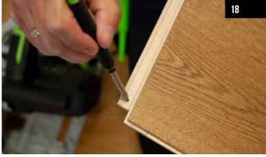
Make sure you cut off the 5Gc short end of the board, the one with the plastic insert, before you draw the cutting.
