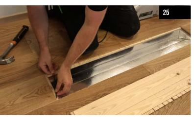
Before fitting the board in the open areas, remove the plastic insert of the 5Gc lock, to make sure you will not to accidentally snap in place.
