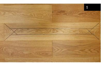
Start by marking the cutting lines on the damaged plank, which should look similar to the above picture (Image 01 and resemble the shape of an envelope).
