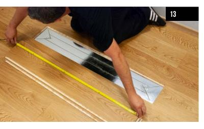
Measure the board and check if it fits in the place of the removed one. It cannot be shorter than the board being replaced.
