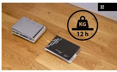
Use a weighted item on the replaced board, i.e., heavy books or other items. Leave weight on the replaced board for 12 hours.
