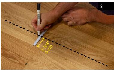
Draw lines with pencil or marker along the long side, approx. 40 mm (1-9/16") from the edge for a wide board 130 mm (5-1/8") or 60 mm (2-3/8") for wider boards.
