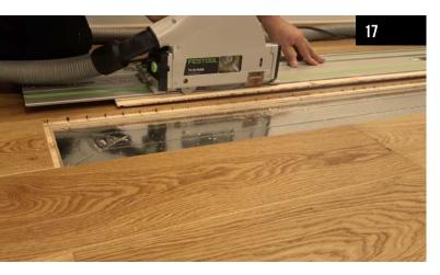
Make a cut on the inverted plank along the marked line so that the new plank can fit in later.
