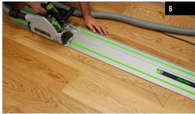
Align the guide rail on the marked line, place the plunge cutter on the guide rail and cut along the drawn line.
