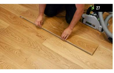
Make an attempt to fit the board. In case the board is too tight of a fit in width or length, correct the new plank with sandpaper or a small plane. If it fits, take it out and put it back in the floor, the previously removed 5Gc insert.
