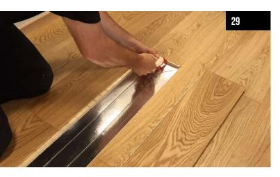
Repeat the operation on the short edge of the board, the one without the 5Gc insert.
