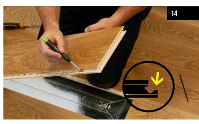
Make sure which profile edger needs to be cut before you draw the cut lines.
