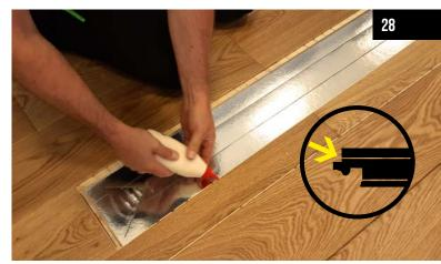
Apply waterproof carpentry glue to the outer part of the long edge of the tongue of the adjacent plank.
