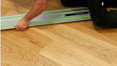
Connect the vertex with the corners of the board being replaced. After the line is drawn, a triangle will be formed. Repeat on the other side.
