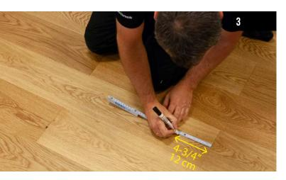
Mark the top of the diagonal lines forming the target triangle, approx. 120 mm (4-3/4") from the short side of the board.
