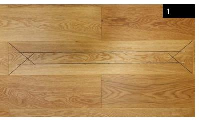
Start by marking the cutting lines on the damaged plank, which should look similar to the above picture (Image 01 and resemble the shape of an envelope).
