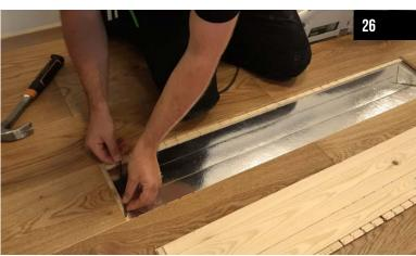
Before fitting the board in the open areas, remove the plastic insert of the 5Gc lock, to make sure you will not to accidentally snap in place.
