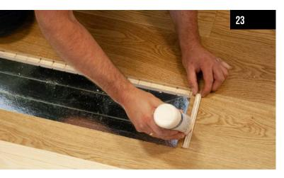
Apply waterproof carpentry glue and attach it under an edge of an adjacent plank.
