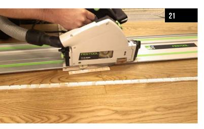
Make a cut along the designated line. Same as in the case of a side joint, this will allow the new board to fit in in place of the board removed. Remove any loose wood fibers and debris from the cutting edge with sandpaper.
