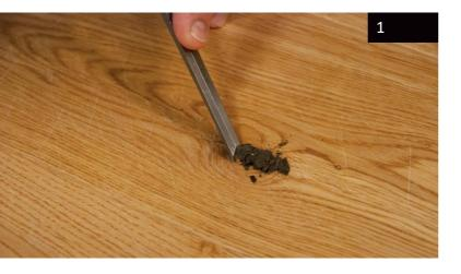
Using a chisel or scrapers, thoroughly clean the damaged area of the joint compound residues or loose wood fibres.
