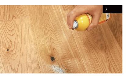
In the case of lacquered floor, the surface must be protected with a sprayable or marker correction lacquer with the appropriate gloss.
