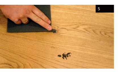
To remove any residual wax, carefully wipe the filling surface with an abrasive pad.
